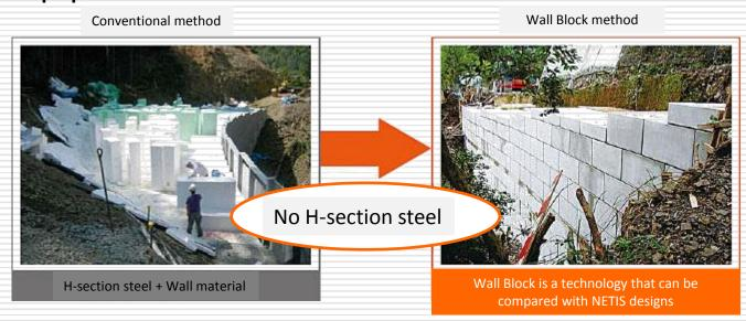
Light: About one-fourth the weight of conventional concrete panels
